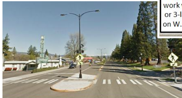
Pedestrian-Activated Crossing in Ashland (Flashing Beacon)
